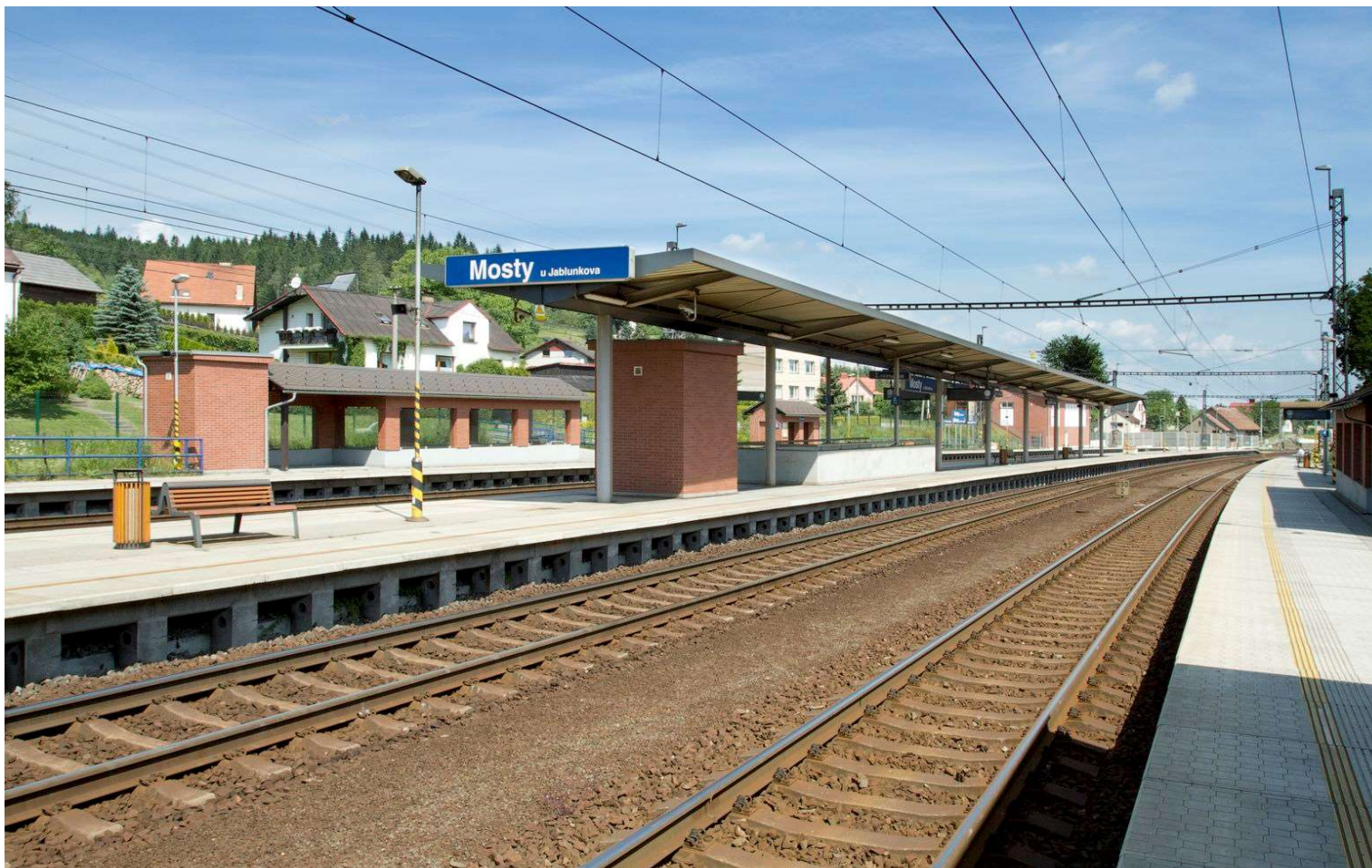
Stanice Mosty u Jablunkova
